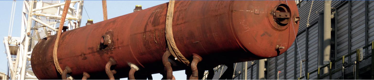
Unit Superheater Engineering (USE) undertook an extremely challenging repair and upgrade of two high pressure steam drums for the HRSG's at a CCGT plant in Runcorn, Cheshire.
